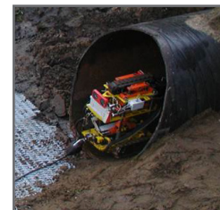
Cut Pipe End
